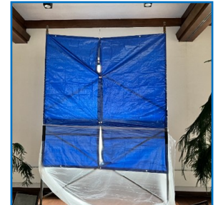
Interior enclosed during window work
